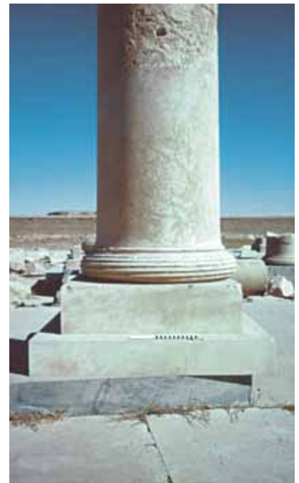
Fig. 16 Detail of a stone column in Palace P. The horizontally fluted torus is carved in one piece with the drum above. Photo: O. Kitson.
