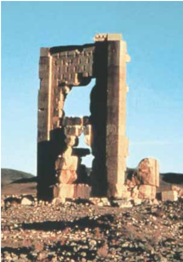
Fig. 17 The Zendān from the west in 1963. Note the remains of the staircase that led to the single immured room nearly eight meters above ground level. Photo: O. Kitson.
